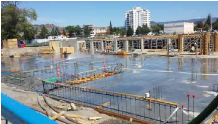
Construction at the Central Green site.
